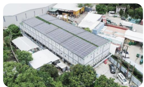
Installation of Solar Panels on the Rooftop of Project Site Office 在地盤寫字樓的屋頂設置太陽能板
