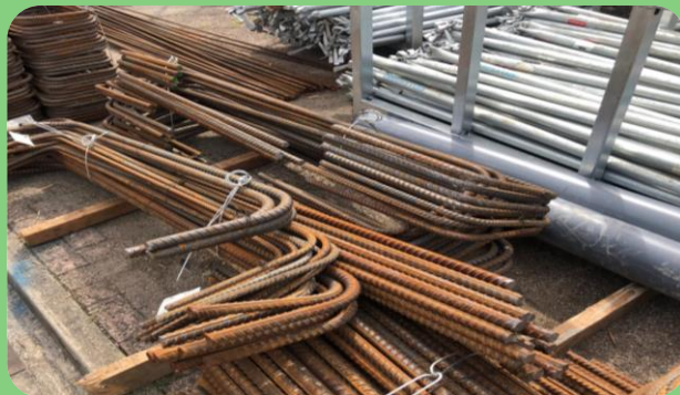
Adoption of Off-site Pre-fabricated Reinforcing Steel Bars 採用場外預製鋼筋組件
